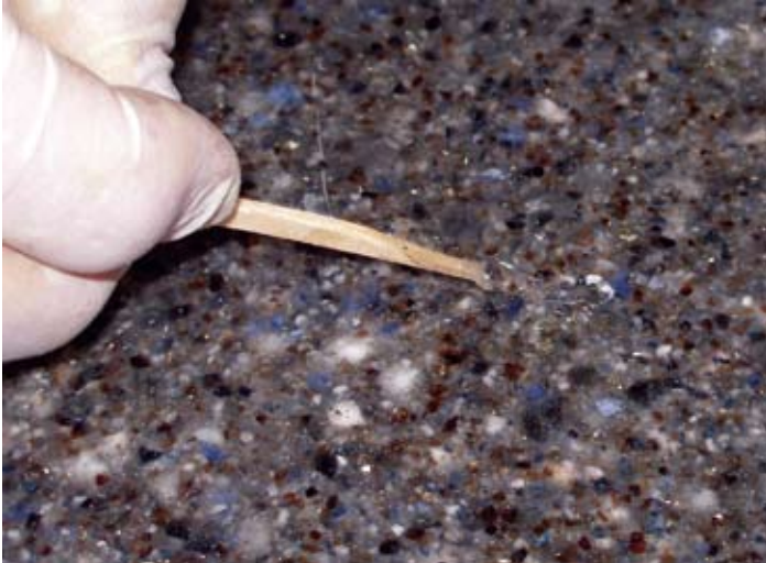
Figure Three: Filling the void carefully and avoiding spilling material on surrounding area.
