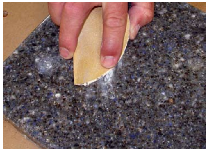
Figure Seven: Sand away excess material that is above or even with gel coat.
